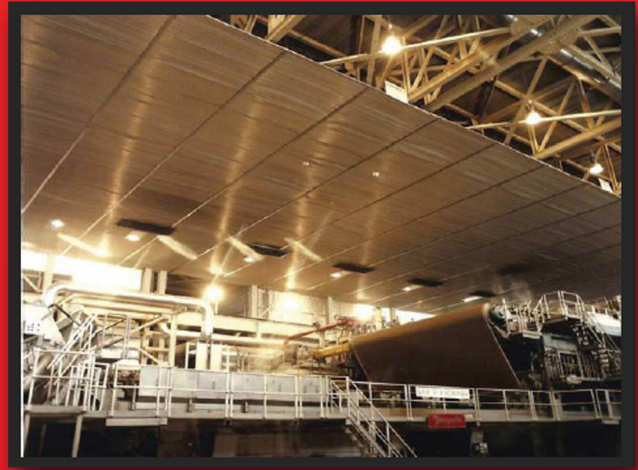
PAPER MACHINE ROOM FALSE CEILING
